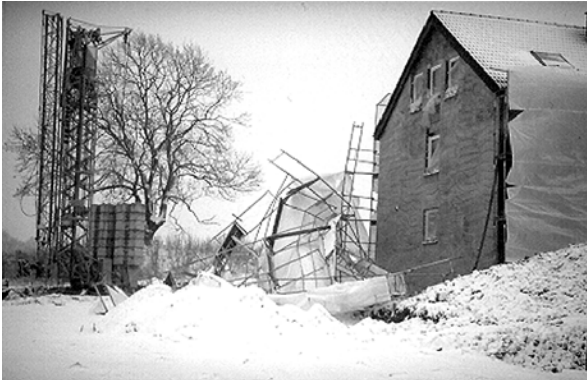
Figure 2 Scaffolding after a winter storm
